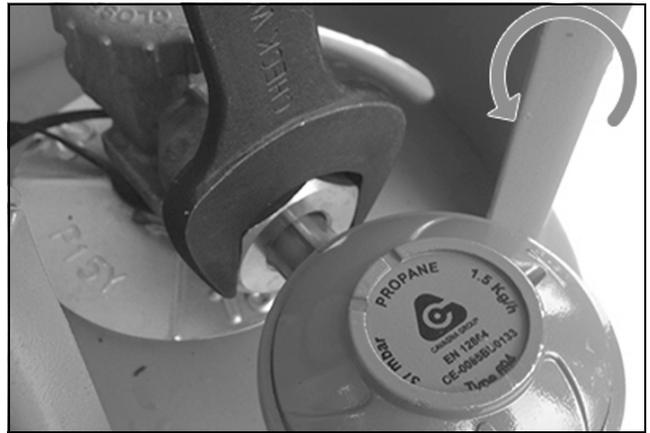
6. Simply turn the valve hand wheel anti-clockwise when you need to start the flow of gas. Ensure that you turn the cylinder off when not in use.
