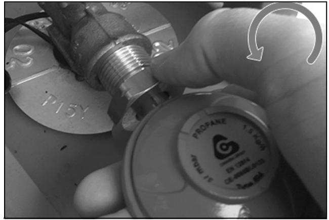
5. Tighten firmly using a gas spanner (or an adjustable spanner), continuing in an anti-clockwise direction.
